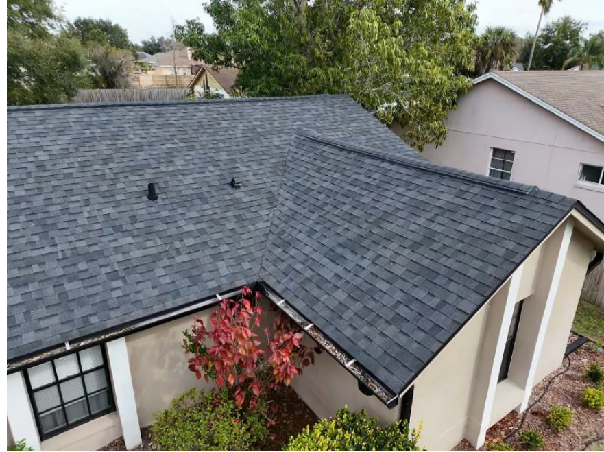
Additional Roof Photo
