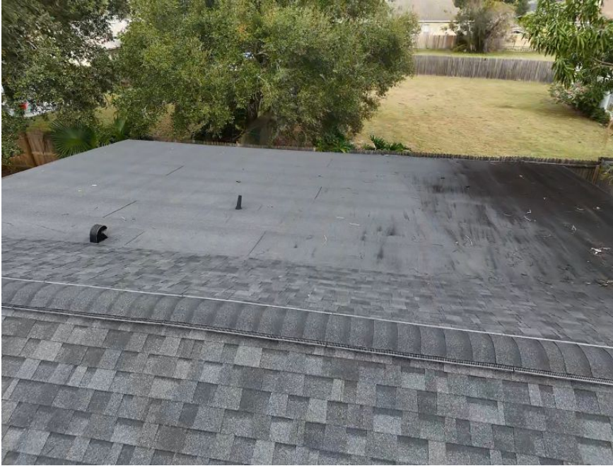
Additional Roof Photo
