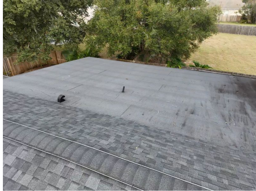
Additional Roof Photo
