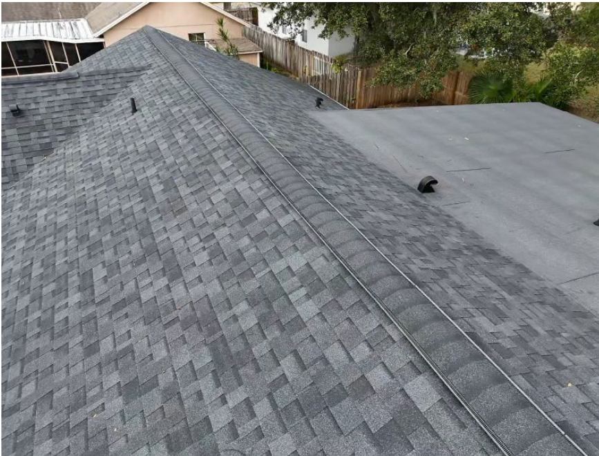
Additional Roof Photo
