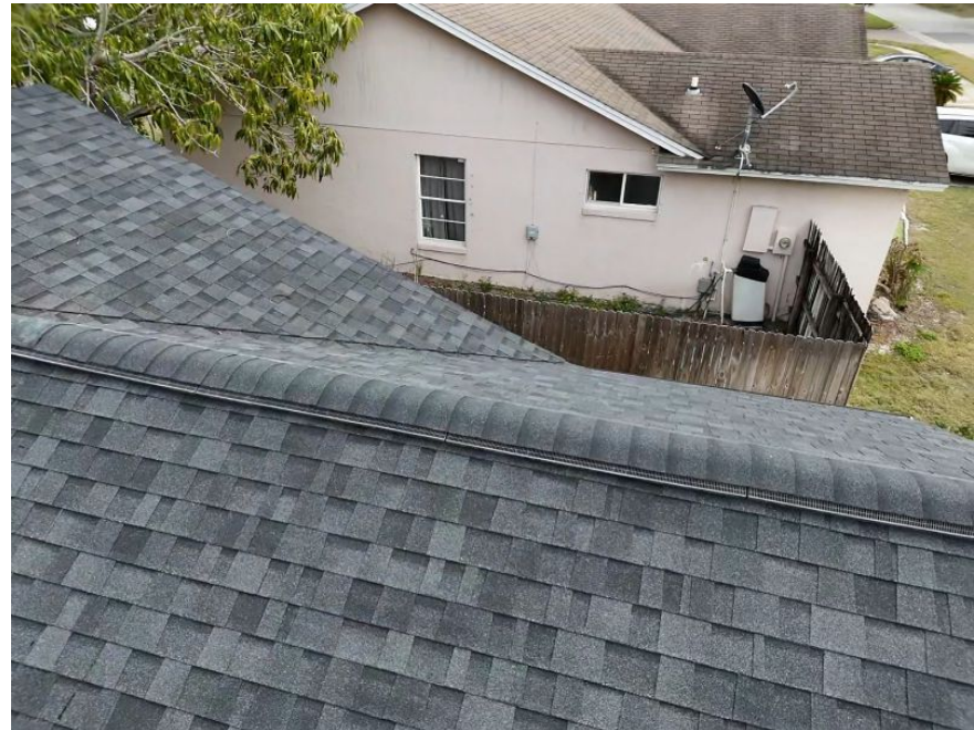
Additional Roof Photo
