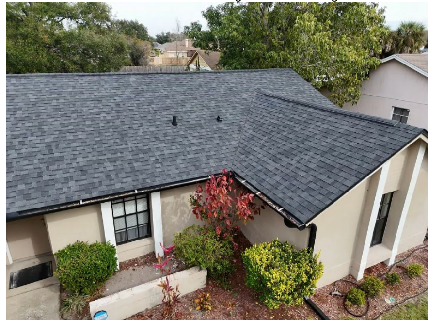
Additional Roof Photo
