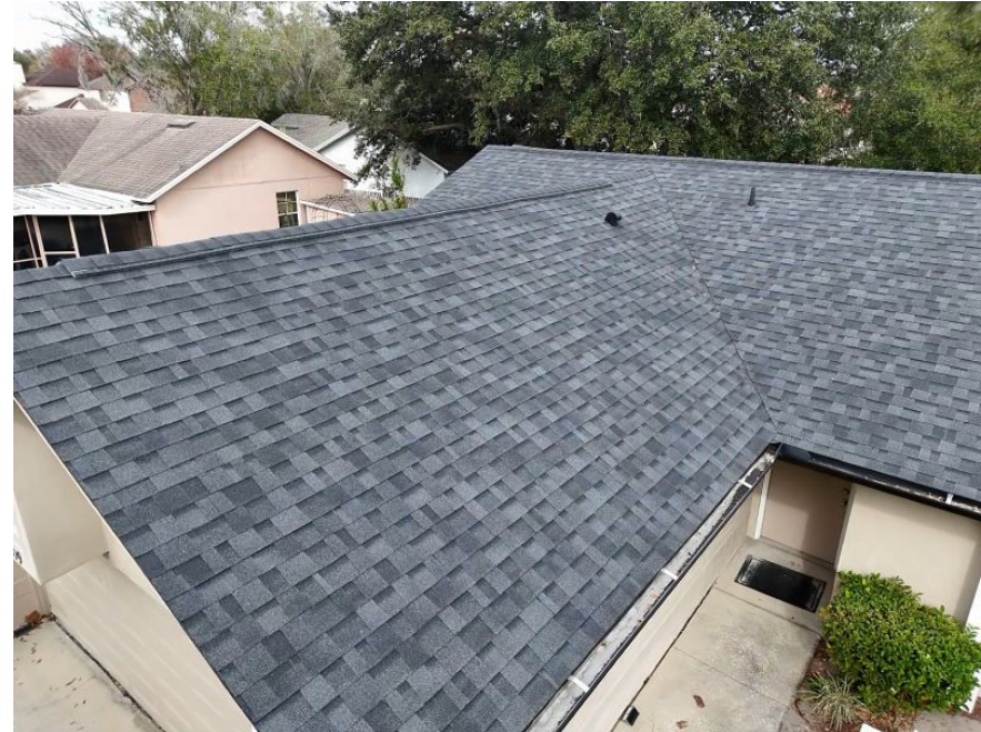
Architectural/Dimensional Shingle Roof Covering
