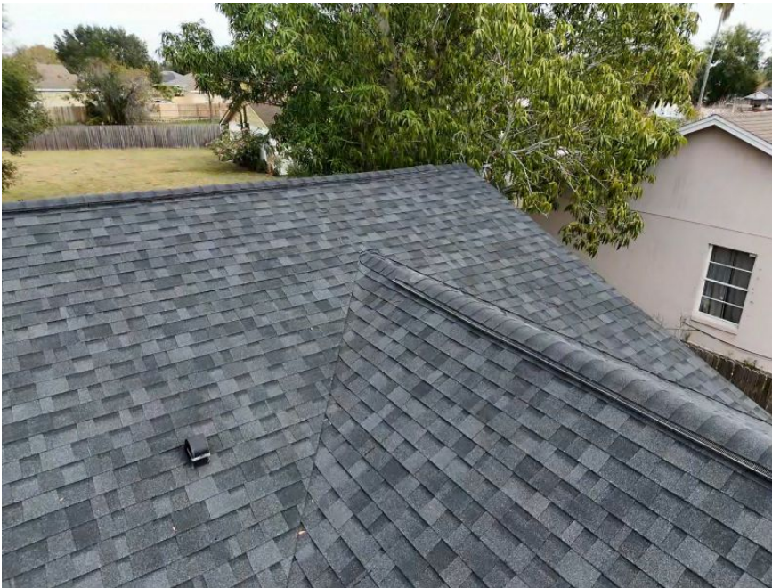
Additional Roof Photo
