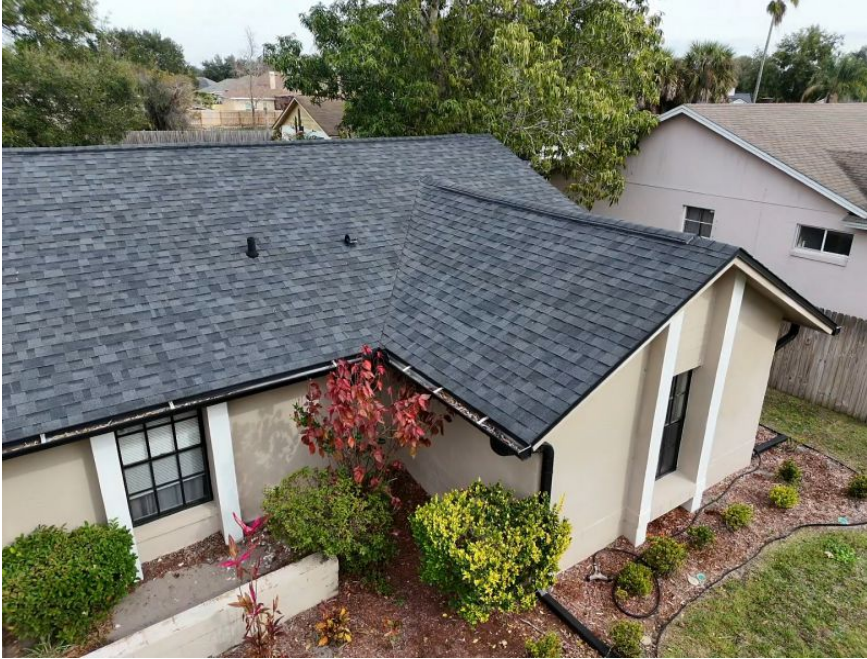
Additional Roof Photo
