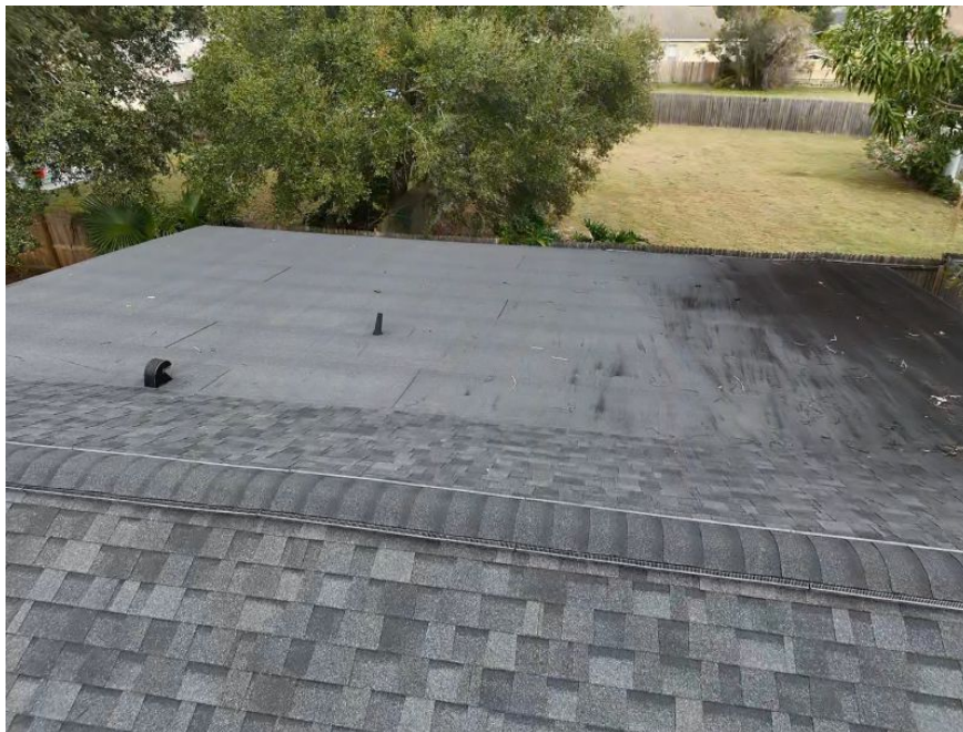
Built-Up/Rolled Asphalt (Sloped) Roof Covering
